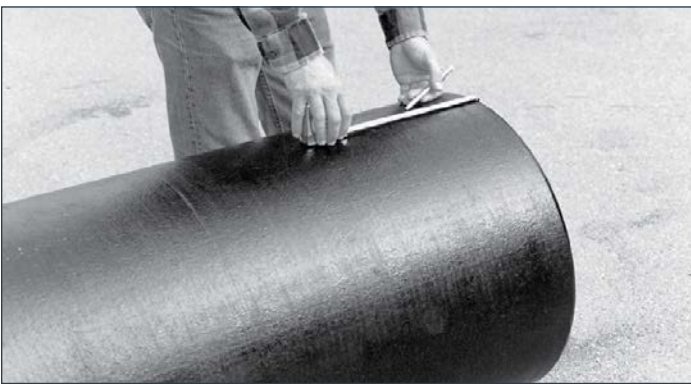
Step 4. Mark the location of the weld-on retainer ring from the cut end of the pipe per the manufacturer's specifications.
