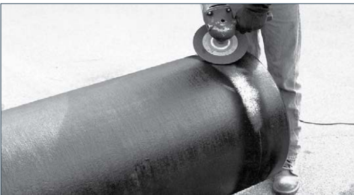
Step 5. Remove the pipe's asphaltic coating on the area where the retainer ring will be welded with a solvent wash or by burning with a torch; then grind the retainer location to bright metal.
